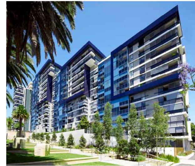
CAMPERDOWN, city quarter - 500+ dwellings - 10-17 storeys 1.7km to subject site
